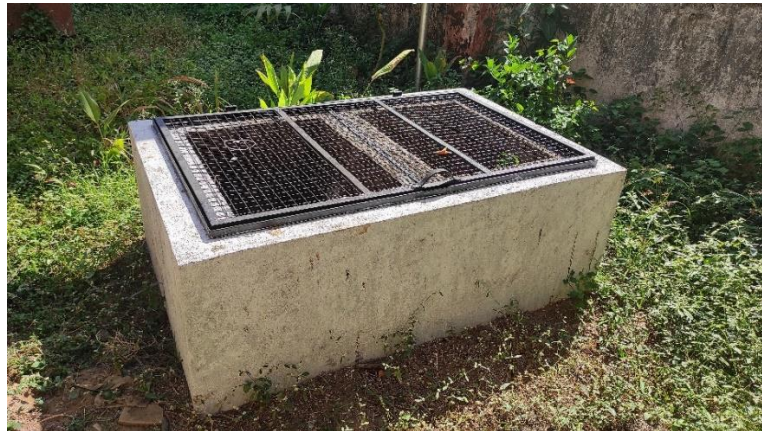
On-site Composting Tank
