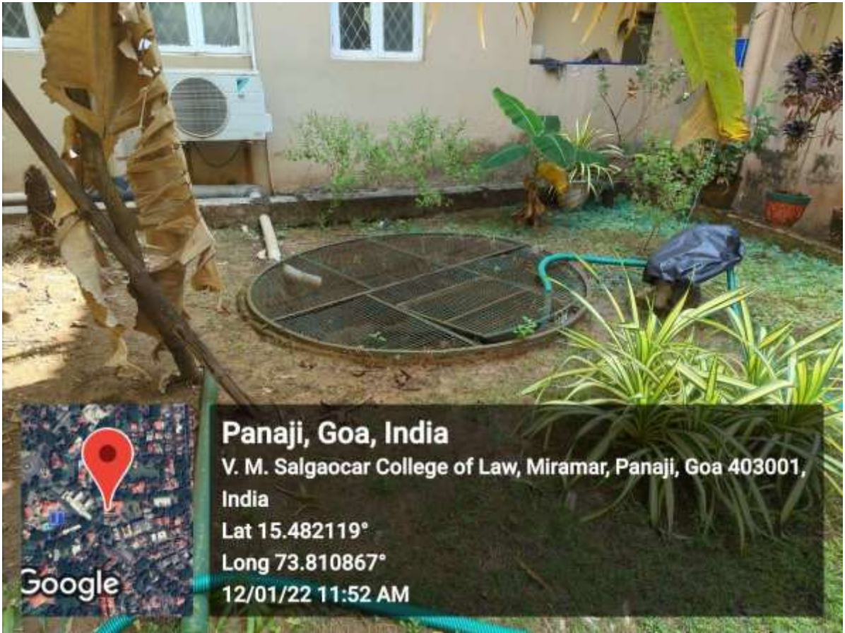
Rooftop water harvesting system
