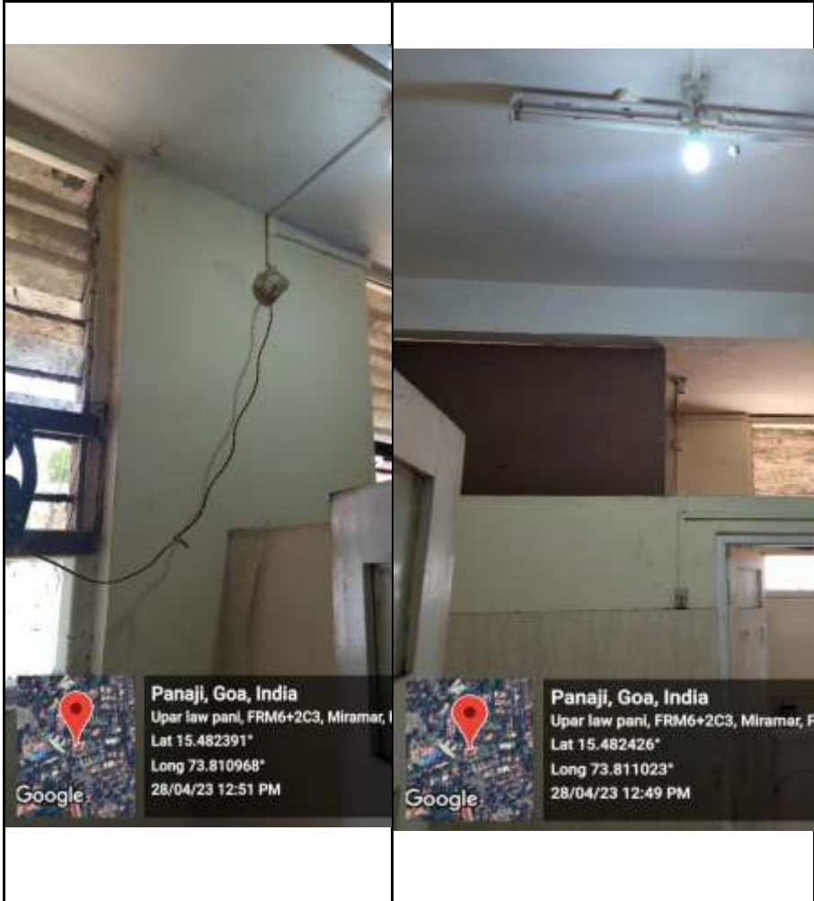
Motion sensors installed in the washrooms for energy saving
