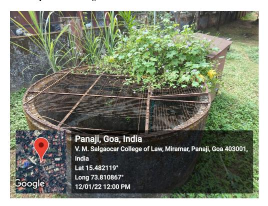
Implementing the 2nd open well recharge system in our college has had several positive impacts. This unit is not connected to rainwater rooftops but exists independently. The system has helped to recharge the groundwater reserves, which has improved the availability of water resources and reduced the risk of water scarcity.
